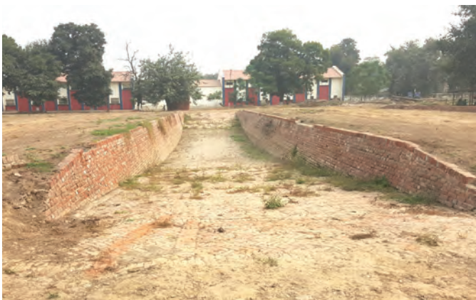
Fig. 1.9(a): Structure of bunker-type silo
